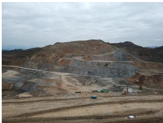
采场南侧边坡
