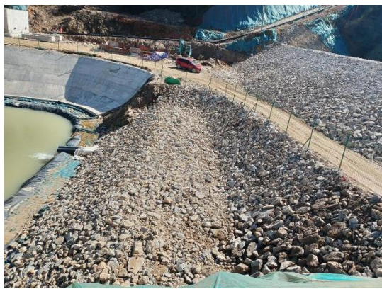
排土场下游拦挡坝
